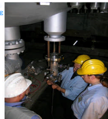
6. E+H Personnel supervision during installation
