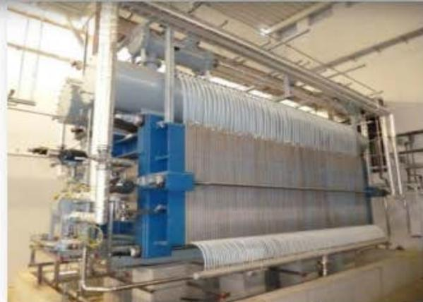
One of three 2MW<sub>el</sub> electrolyzers
