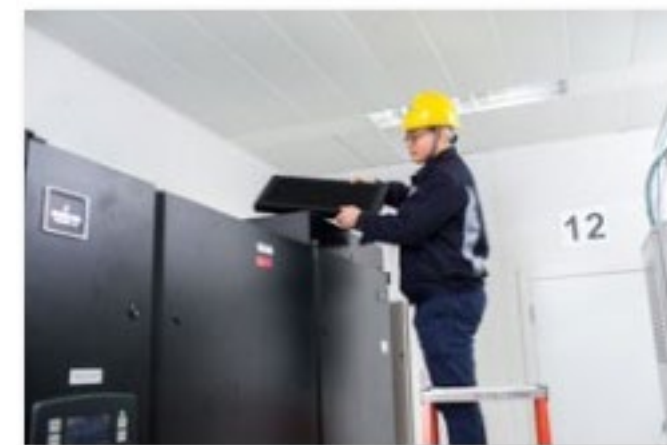
Figure 5 - Once the honeycomb modules are installed, no further maintenance is needed. The filters run for up to five years before they have to be changed.
