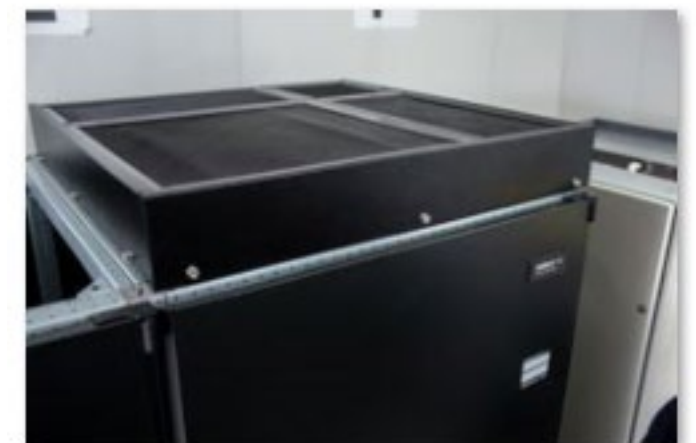
Figure 2 - Honeycomb modules: walls made of activated carbon powder, which are held in shape by ceramic binders allow a high flow velocity.
