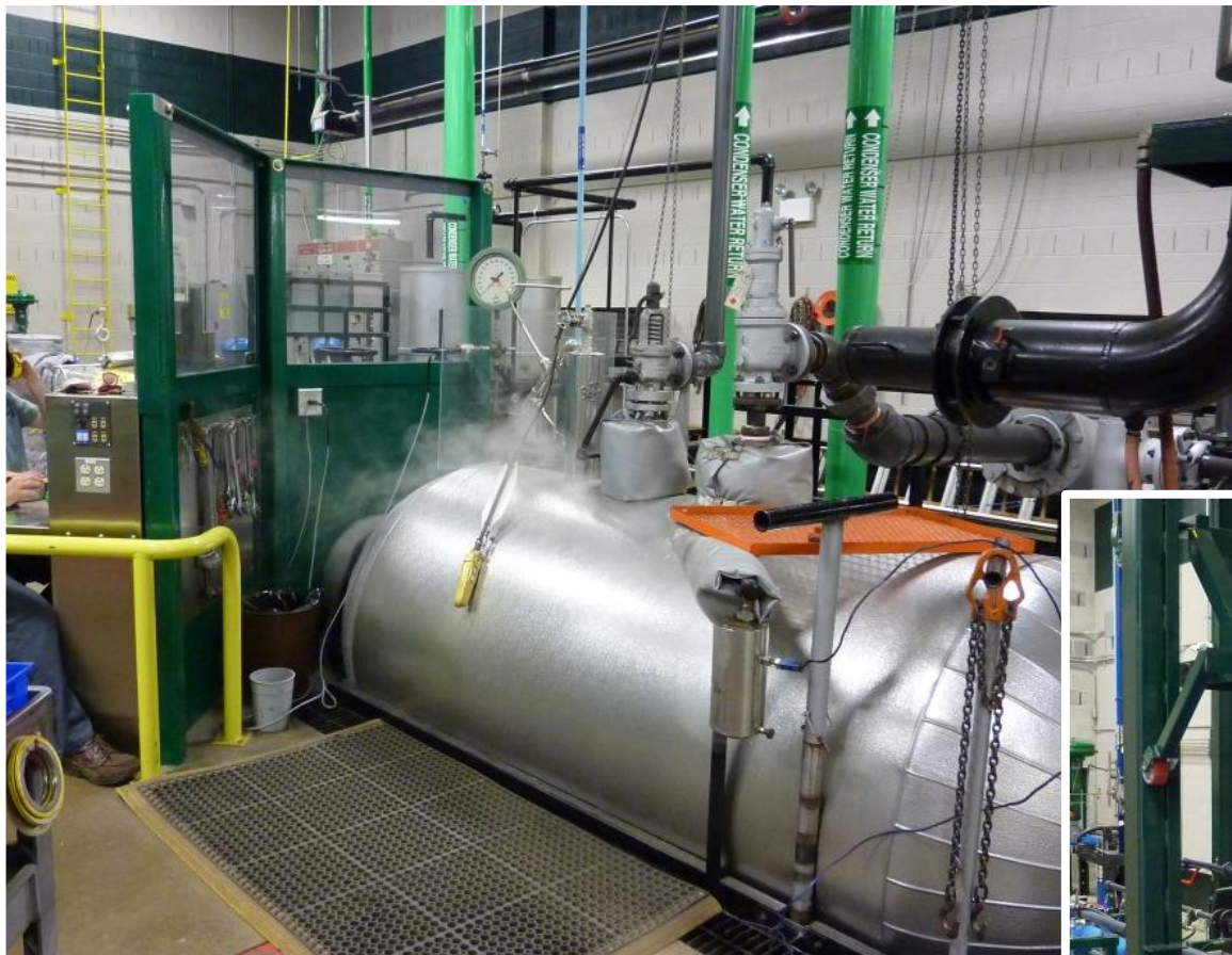
DN 2" J 3" during testing with steam
